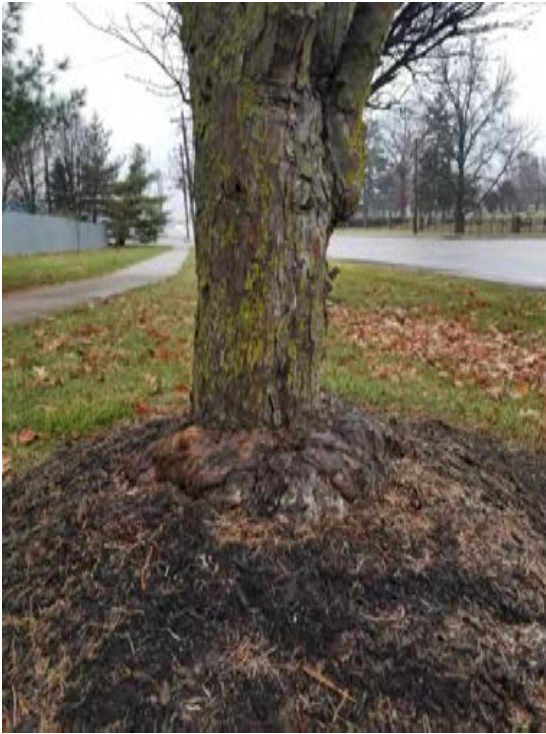
Significant mechanical damage around root collar, including decay and trunk splitting further above ground.
